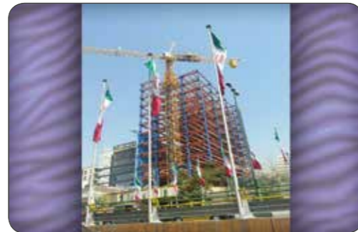
Mirdamad Steel Structure
