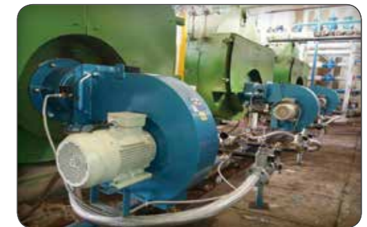
Three Gas burner Type: MFG500 Capacity: 3500000 kcal/h Project name: commercial complex Project location: Mah shahr
