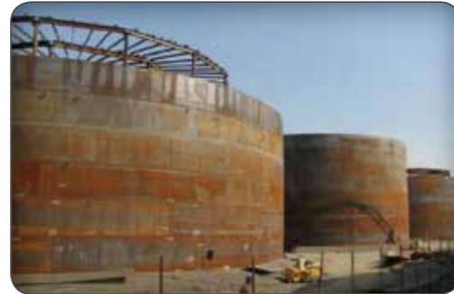
Atmospheric Storage Tank
