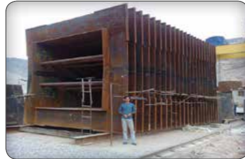
Hydromechanical and electrical equipment of Gotvand Dam
