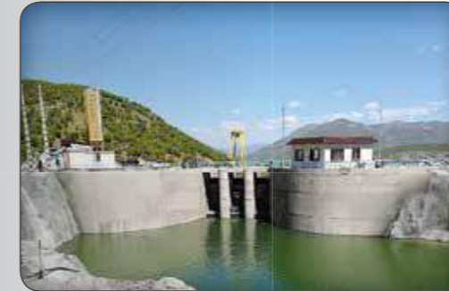
Hydromechanical and electrical equipment of Abas abad Dam
