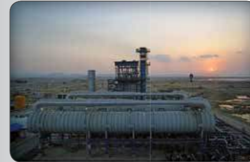
Thermal Desalination Plant(MED-TVtype) Qeshm water and power plant
