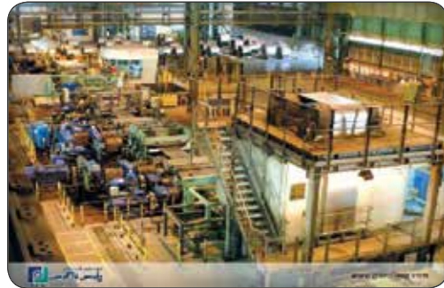
Steel Coil Inspection Lines (EPC Contract)
