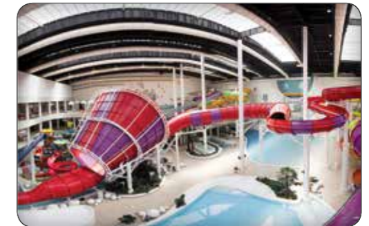
Heat Exchanger, Boiler & Other Boiler Room Accessories Opark Water Park (Tehran)
