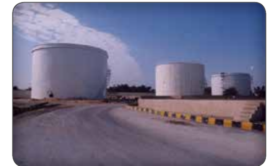
E.P.C. Construction & Installation of 6 Sets Storage Tanks- Zahedan, Yazd & Rafsanjan
