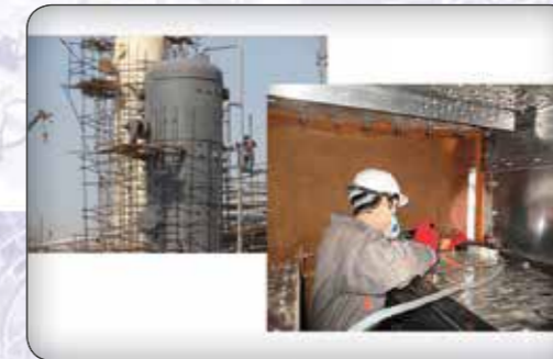
Installation and Installation supervision services
