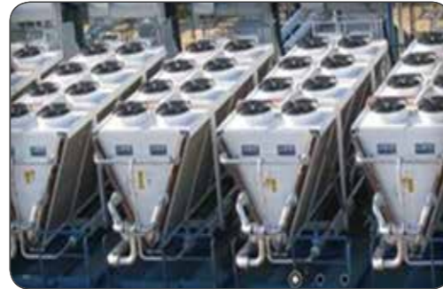
Industrial Dry Coolers
