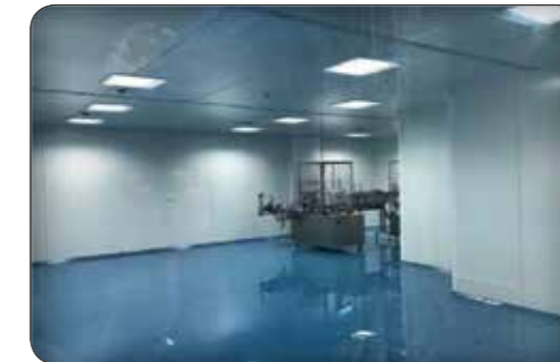
Design and Installation of Clean Room
