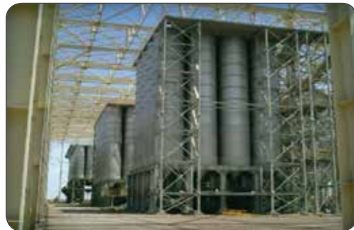
Silo / Duct Apadana Ceram Co.
