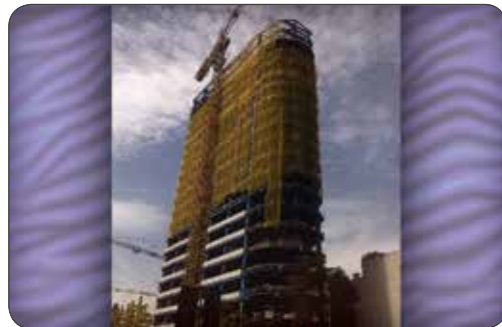
Construction of steel structure, Royal Building project
