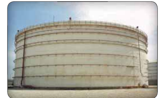
Fixed & Floating Roof Storage Tanks (Manufacturing of Floating Roof Storage Tanks for Boali Sina Petrochemical Plant)
