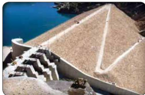
Masjed Soleiman Dam and Power Plant
