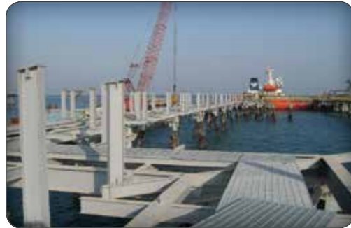
Renew & Repair Project of Kharg Preparatory Harbor- Kharg Island
