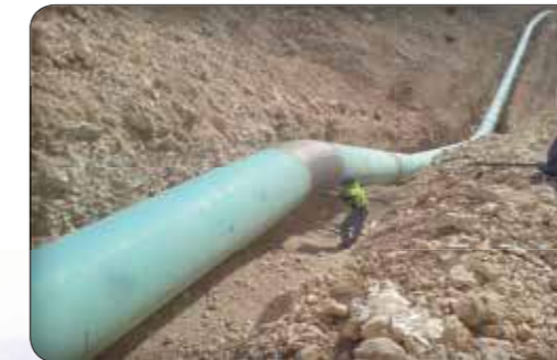
On-Site Field-Joint Coatings and Rehabilitation
