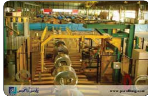
Steel Coil Packing Line (EPC Contract)
