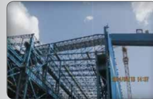
Construction of Platforms, Structures & Handrails (Jahan Ara Arvand Steel (AJS) Factory)
