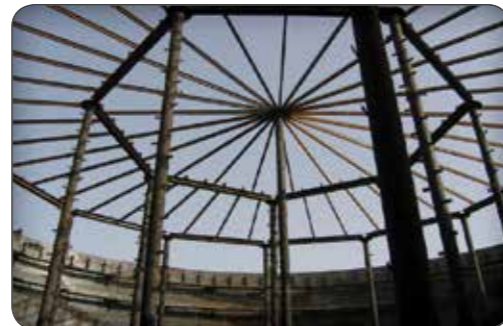
Construction of 2820 m3 Floating Roof Tanks- Kermanshah, Eslamabad & Ghasreshirin
