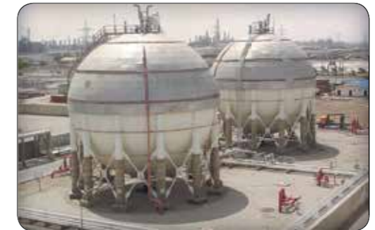
Spherical & Double Wall Tanks (Manufacturing of Spherical Tanks for Ilam Gas Refinery)
