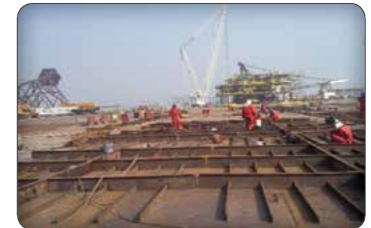
Two Pantan Jetty Construction Project at Choebdeh & Arvandkenar- Choebdeh
