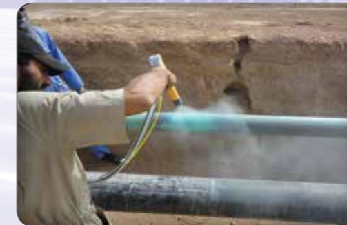
On-Site Field-Joint Coatings and Rehabilitation
