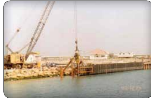
Breakwater & Wharf Construction- Sirri Island
