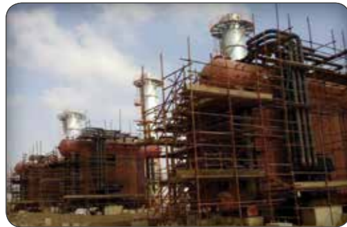
Steam Water Tube Boilers: Up to 600 Tons per Hour under License of Eck Rohr Kessel GMBH Germany
