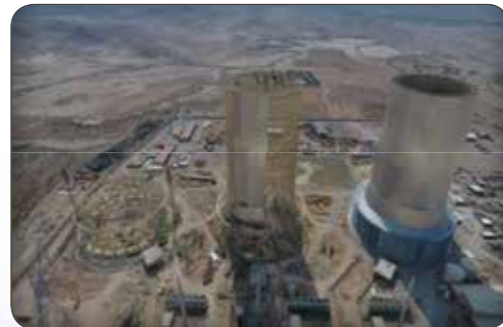
HELER -Dry Cooling Tower Jahrom Combined Cycle Power Plant
