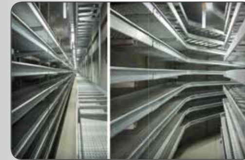
Production of Steel Production Lines Cable Trays and Ladders (Isfahan Zobahan Saba Steel Development Plan)
