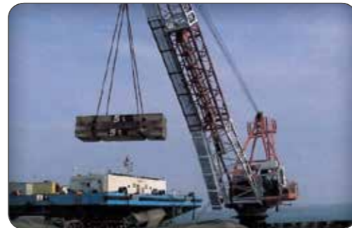
Construction of Marine Pedestal Crane- South Pars Phases 4 & 5
