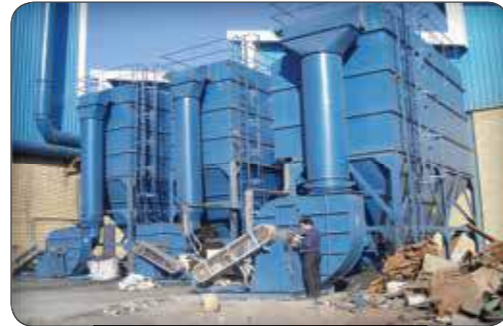
BAG FILTERS (Jet - Pulse) Chadormalu Direct Reduction & Steel Making Plant Sangan Pelletizing Plant 1&2. Abade, Jovein, Delijan Cement Co.
