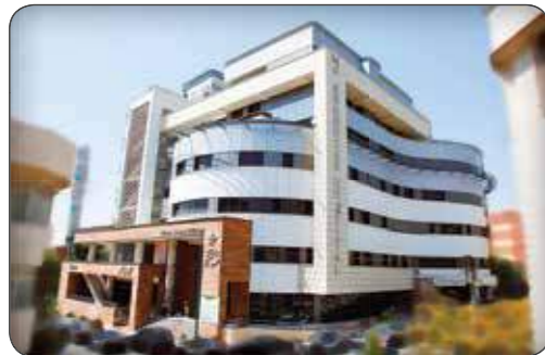
Vertical Steam Boiler Moheb Kosar Hospital
