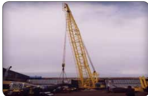
Construction of Marine Pedestal Crane- Khazar Semi- Sub Drilling Unit
