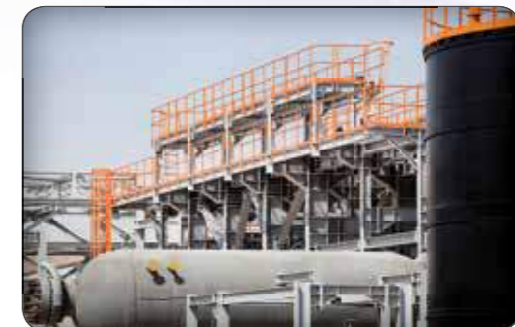
Fabrication and installation of steel structures of Kermanshah petrochemical
