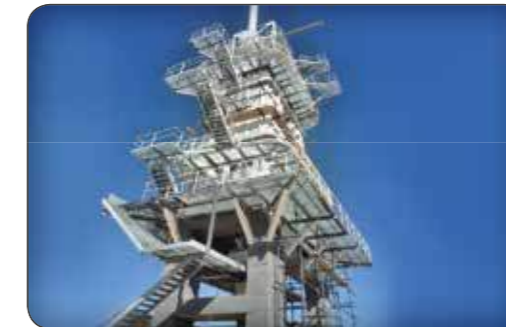
Parallel Flow Regenerative Shaft yazd
