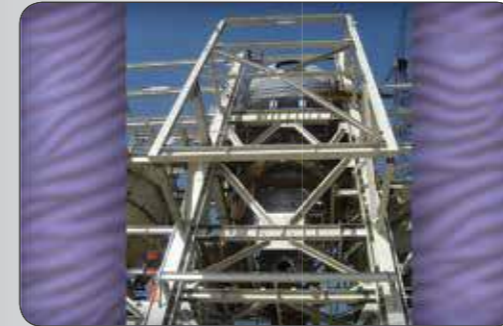
Industrial Steel Structure
