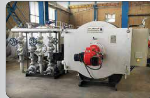
Gas-oil burner Capacity: 800000 kcal/h Type: MFL100-100 On hot furnace Project location: Coveit Company: KMB
