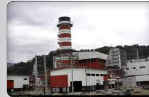
Domestic Hot Water, Boiler & Other Boiler Room Accessories West Mazandaran Combined Cycle Power Plant
