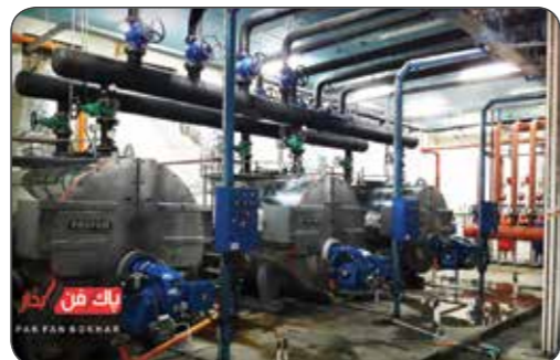
Reverse flame hot water boiler
