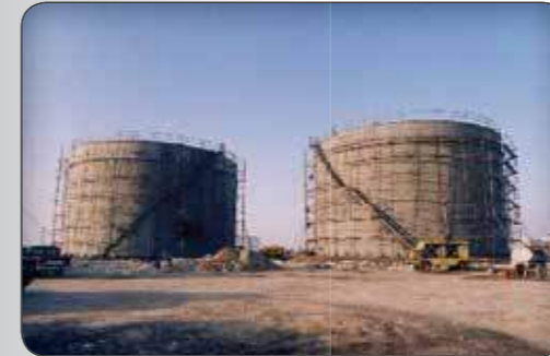
E.P.C. Construction of 5000 m3 Potable Water Storage Tanks- Lavan Island
