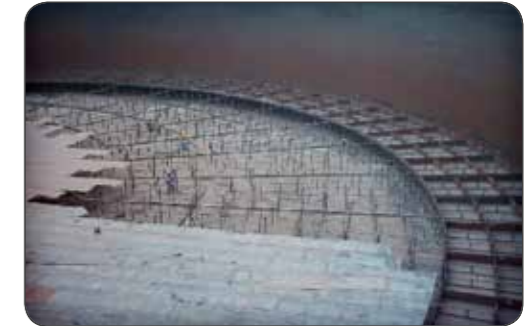
Complete Repair of 1 Million BBL No. 36 Storage Tank- Kharg Island
