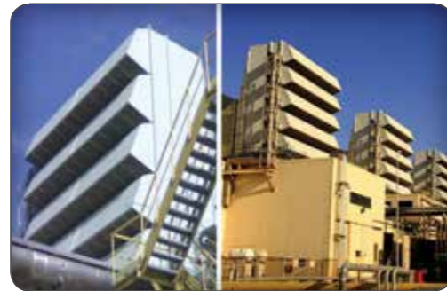
Construction of V94.2 Gas Turbine pre-filter units (Turbine Engineering & Manufacturing Company (TUGA))
