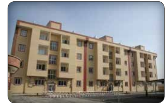
Construction of Two Sets of Staff Resorts of Kharg Petrochemical Co.
