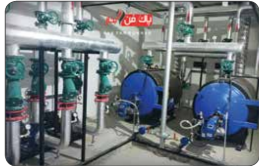
Three pass dry back steam boiler
