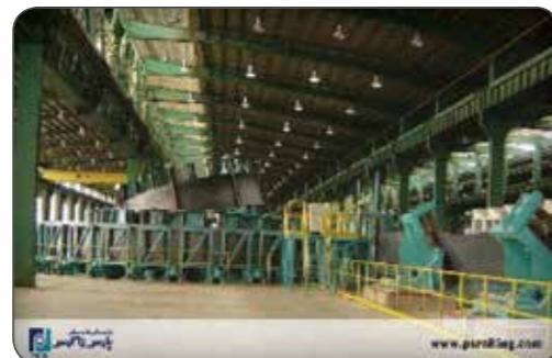
ERW (Electric Resistance Welding) Steel Tube Mill
