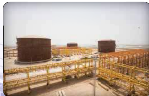
Fabrication of steel structures of Bid Boland Mahshahr plant
