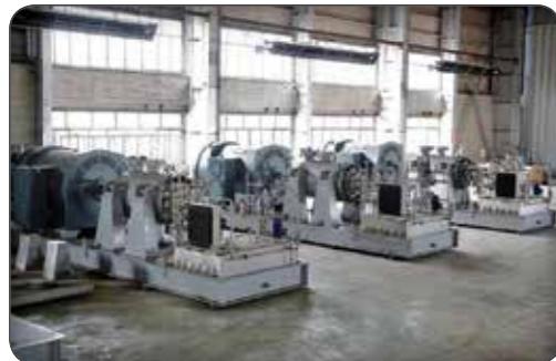
Naein- Kashan- Rey Pipelien Project
